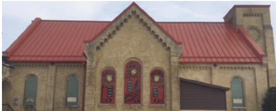
DYNA-GUARD installed on roof
