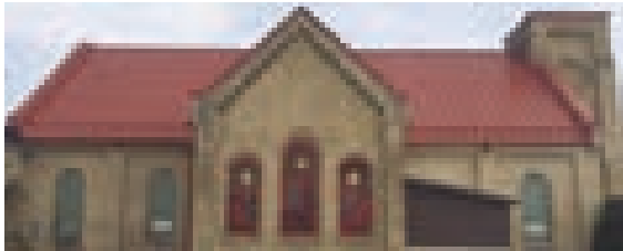
DYNA-GUARD installed on roof
